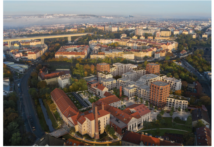
Figure 12 Bird's eye view of the regenerated brewery site towards the northwest, source: Penta Real Estate, 2023
